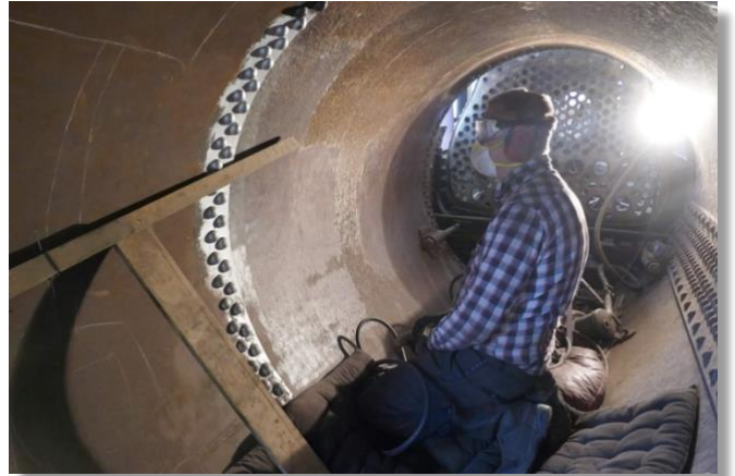
Dick admiring his handiwork - or maybe just tired? You can see the improvement the needle guns makes to the surface.
