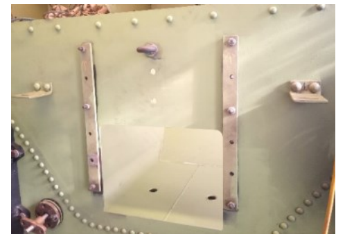
Coal door slides in place.
